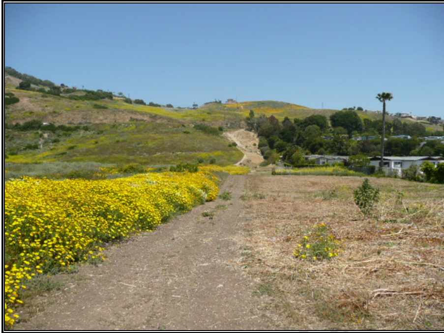
Photo: View north toward the tunnel alignment and 100' easement, cut and cover area.
